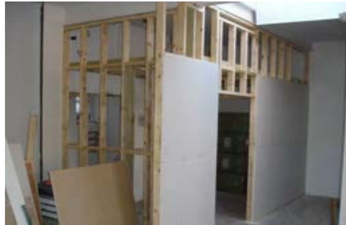
Internal partition frames & walls
