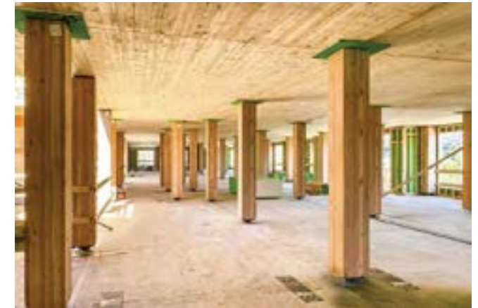
Mass Engineered Timber (CLT & Glulam) – columns & floors
